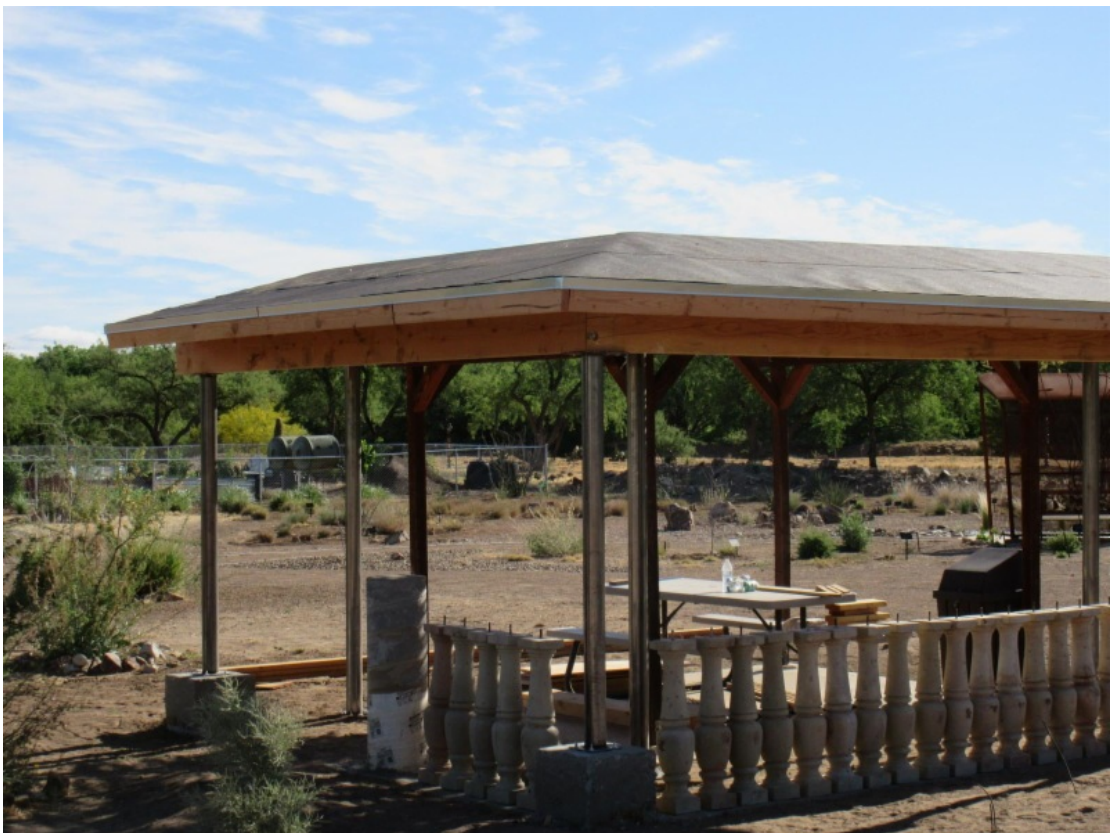
Ramada renovation continues at Desert Meadows Park Chuck Parsons
